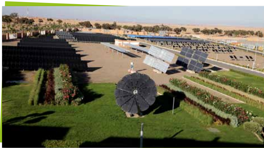
Green Energy Park, Ben Gherir, Morocco
